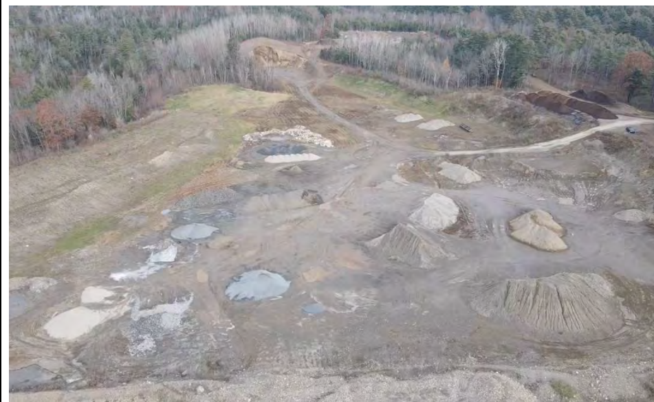
Photo 2 – Drone photograph showing existing conditions within gravel pit. Project proposed to be located within gravel pit.
