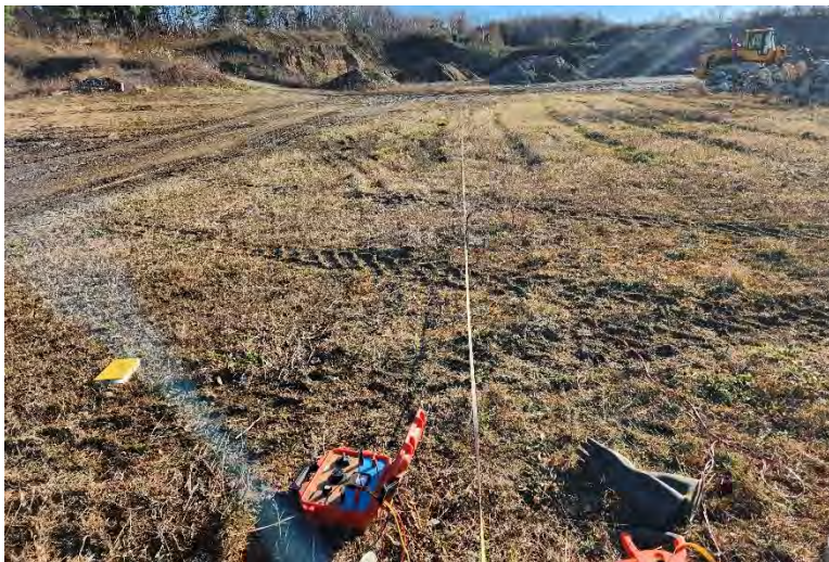
Resistivity Testing near Transformer Pad (Test 1A S-N)
