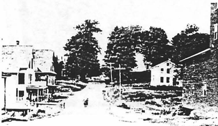
After the fire; Frank Doe's store 1st on left, Dinsmore house and mill on right
